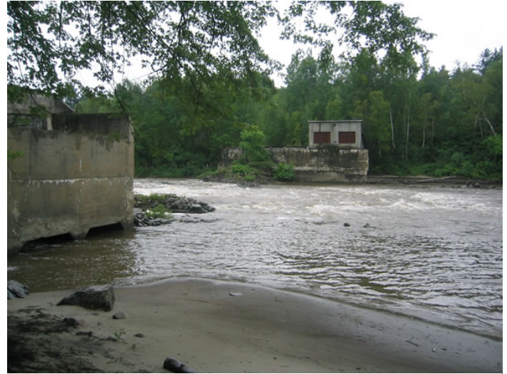
The breached Wyoming Dam site on the Connecticut River.
